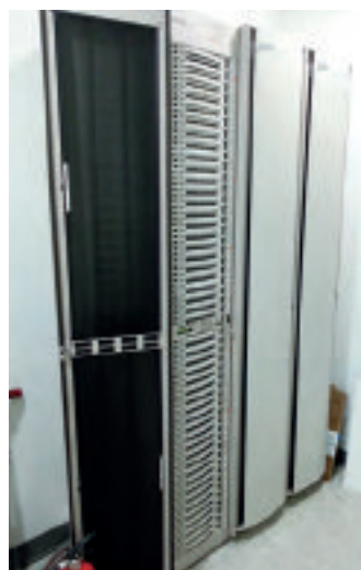
John Black's ETC Sensor3 dimming racks
