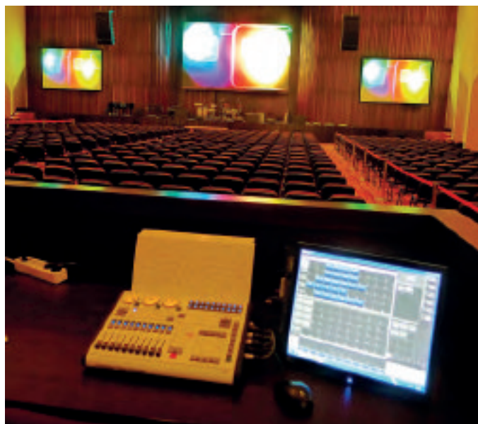
An Avolites Titan Mobile control surface and software manages the lighting at GBI Gilgal
